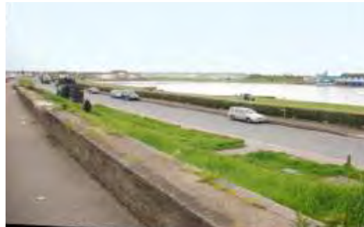
Wharf Road embankment and Hove Lagoon from Kingsway
