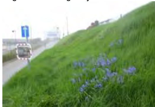
Basin Road North embankment
