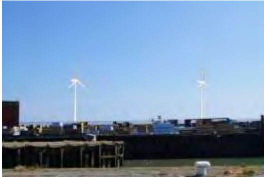
Wind turbines at Outer Layby
